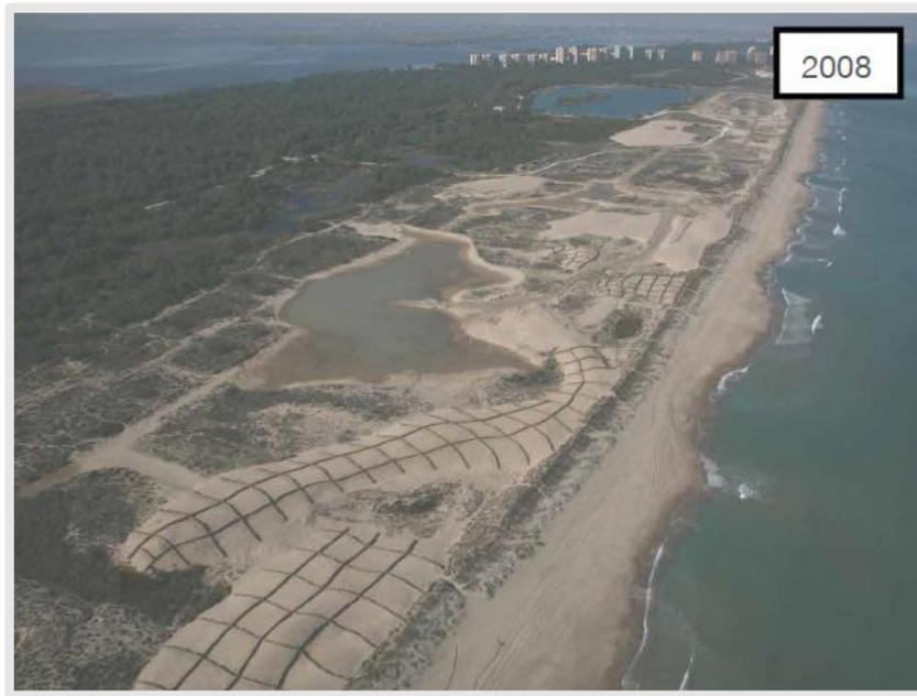
*2008. During the LIFE ENEBRO project: North Malladeta and Brava beaches. The dunes with palisades stand out, recently repopulated with vegetation, and the craters from which part of the sand has been extracted. The first front dune is completely restored.*
