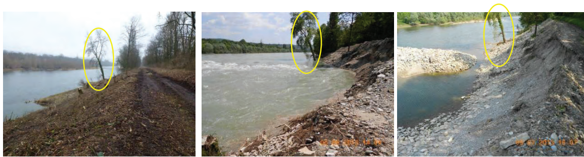
Figure 4: Upstream part of the pilot site of controlled erosion before (left), during (middle) and after (right) the flood.
