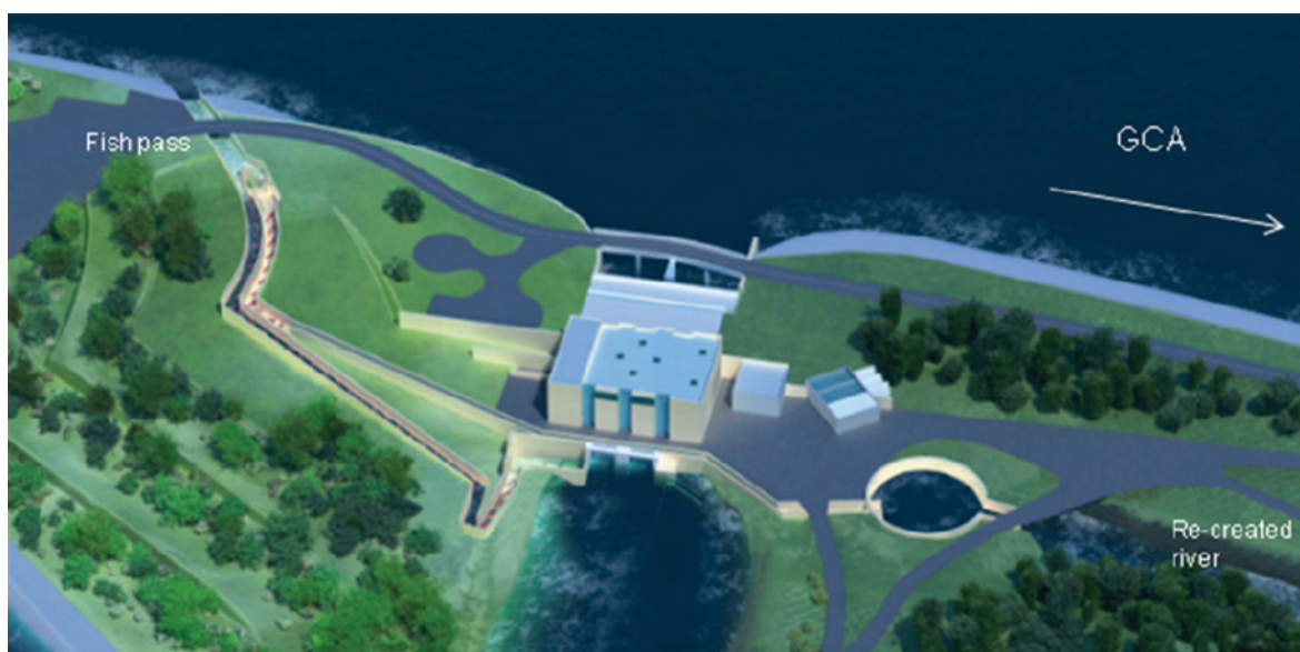
Figure 10: 3D view of the new hydropower plant B with the fish pass and the upstream part of the new river, which is supplied in water through the fish pass and the plant.
