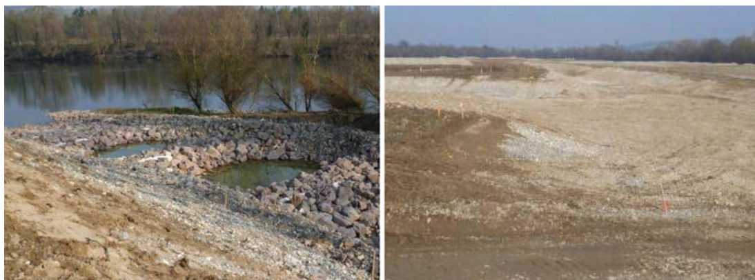
Figure 8: connection between the recreated river and the Old Rhine where the flow will be 5 \text{ m}^3/\text{s} (left) and levelling works in the field: see the separation in 2 arms of the future river. Work is in hand (mars 2014).
