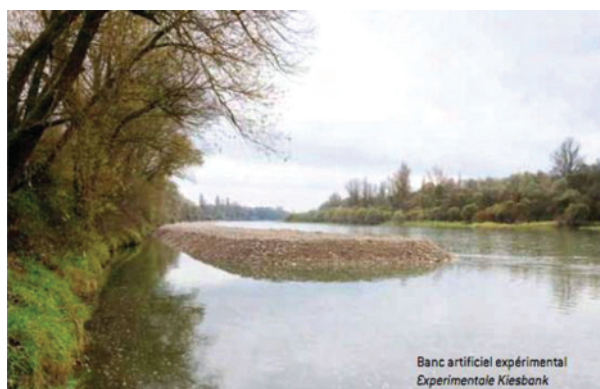
Figure 5: experimental input of sediment excavated from the right bank of the Old Rhine (Interreg project, 2009-2012) (source : Region Alsace).
