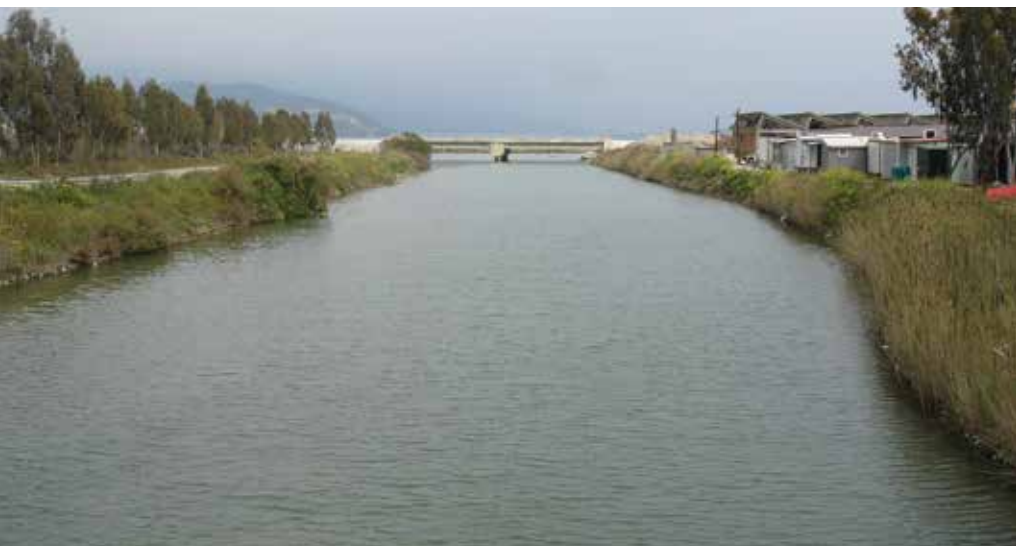
Figure 3.47: In the 1960s, several studies recommended flood control constructions and a drainage network, which emptied Lake Karla's water into the Pagasitikos Gulf via a drainage channel (pictured)
