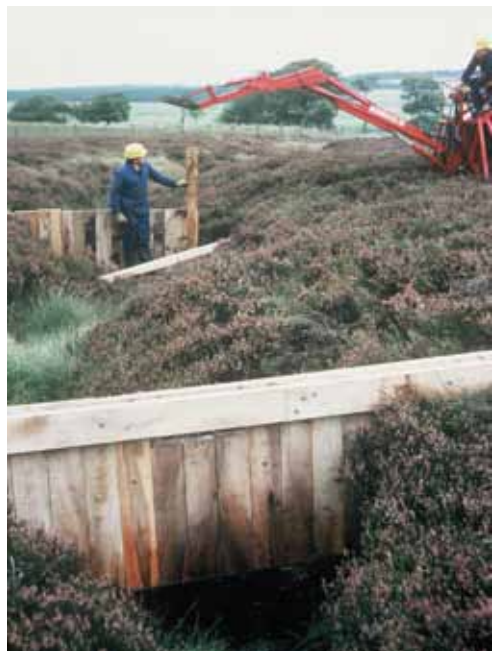
Ditch blocking 1989 © A Panter, SNH
