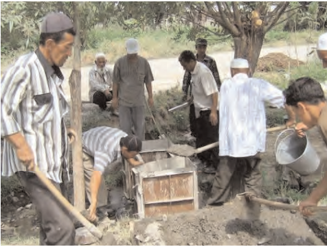
Figure 15. Construction of water metering devices at the WUA level, Kyrgyzstan
