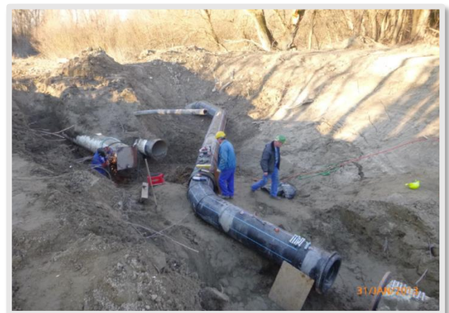
Work on water pipes – Source: WWF
