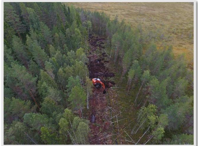
Excavator filling in the drainage ditch in forest-covered mire in North Karelia 2017 © Metsähallitus/M.SIMILA
