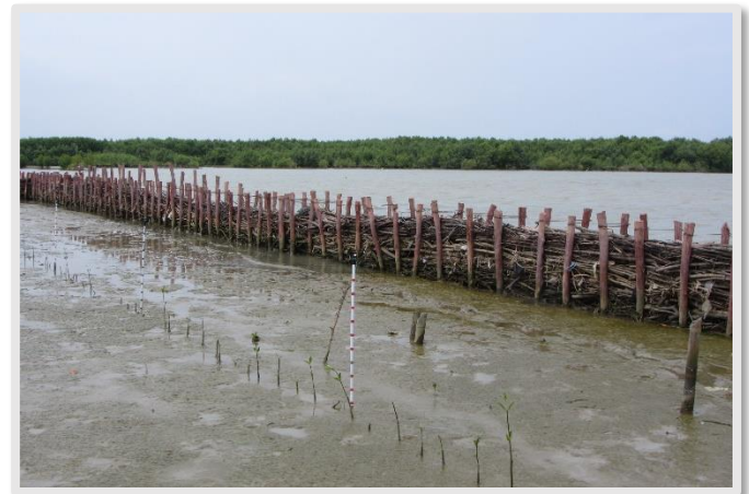
Sediment accumulating inside the permeable dams © TONNEJICK F.
