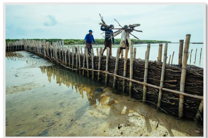
Community involvement in the construction work © Boskalis
