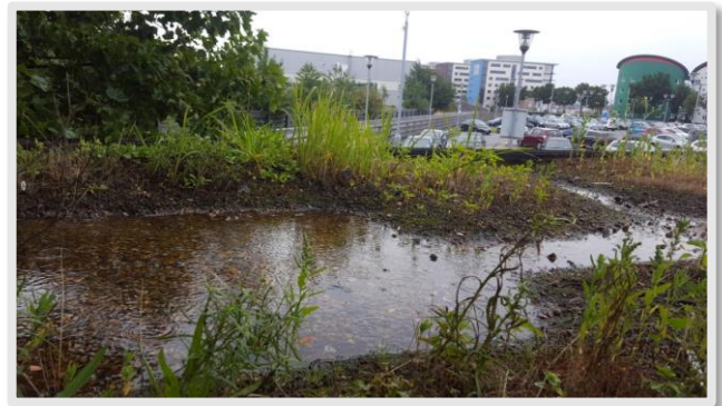
Ephemeral wetland green roof during summer rain event - University of East London Docklands Campus, London, UK. (©UEL SRI)
