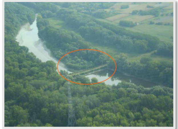
The rock-fill dam – Source: WWF
